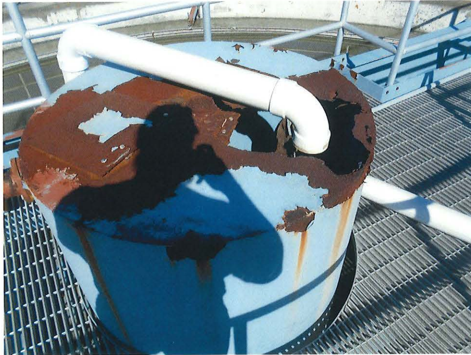
Damaged Imhoff tank cone and temporary scum piping.
