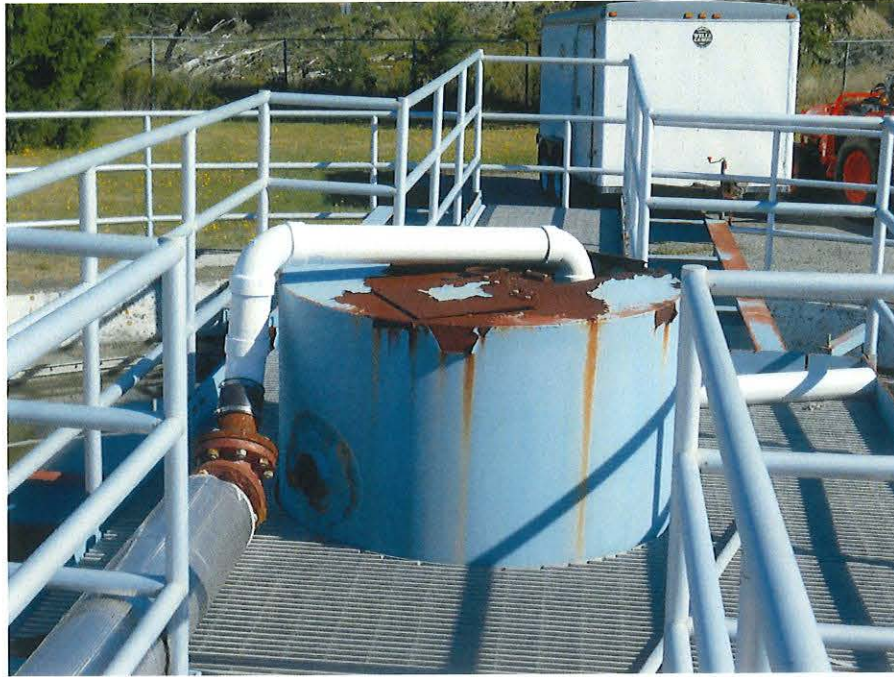
Damaged Imhoff tank cone and temporary scum piping.
