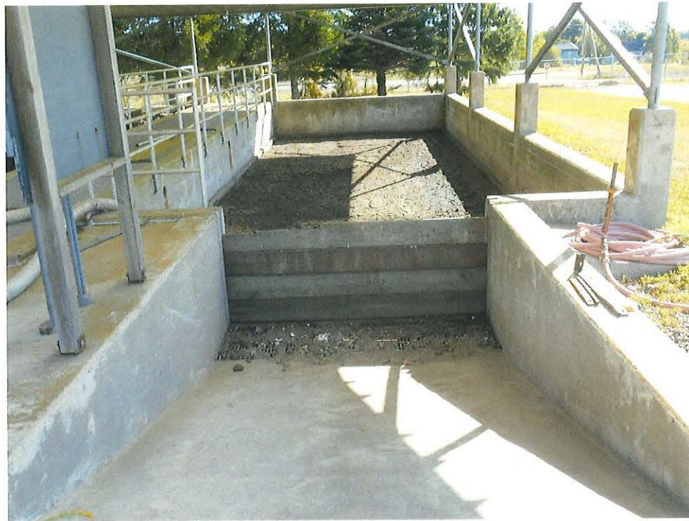
Existing Sludge Drying Beds
