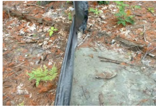
Collected sediments should be removed when one-half the height of the barrier is filled.
