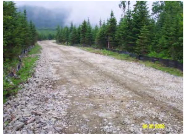
Good road surface and base material contains gravel, sand, and a few fines. Gravel and sand in the subbase provide strength and drainage.
