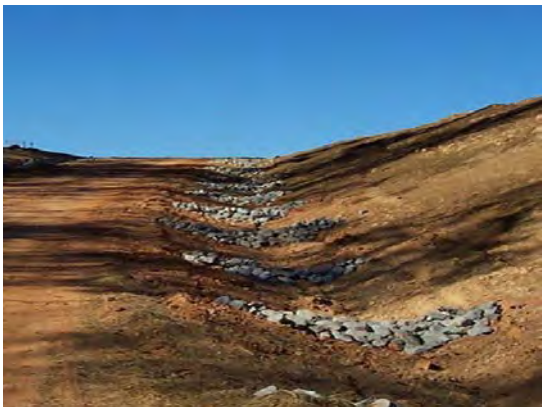
Any erosion downgradient or around the edges of a sediment barrier or check dam should be corrected immediately.
