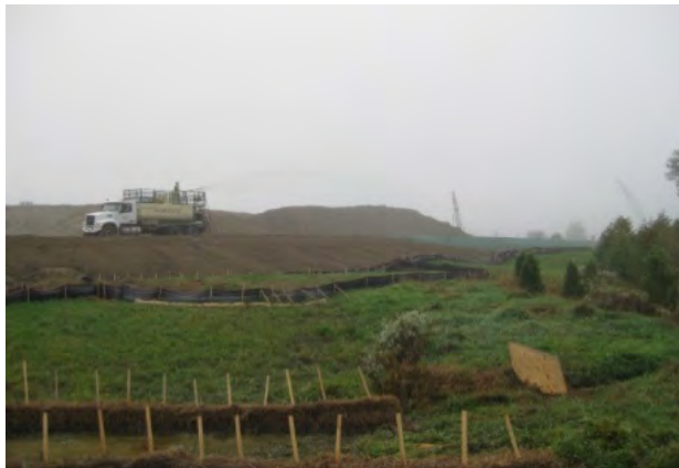
When hydroseeding, apply the seeds uniformly and per applicator's guidance (10% increase in seeding rate is recommended).
