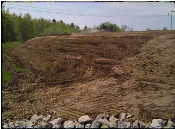
Soft sedimentary rock can be modified to create a surface for vegetation growth when the rock is rippable and can be shelved. The shelves will hold moisture, seed, and mulch.
