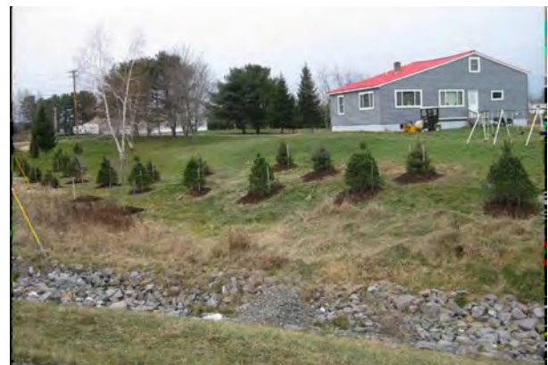
A created buffer should also be stabilized with seeding and mulch.
