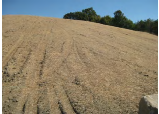
Divert clean water away from the immediate area and disperse to an undisturbed area to reduce erosion
