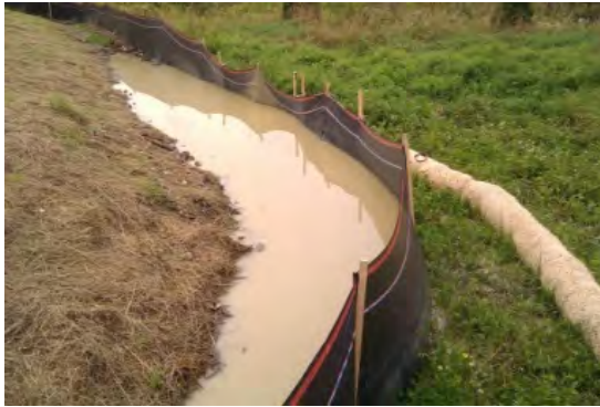
Sediment barriers should be inspected and repaired before, during, and after each rain event.
