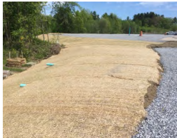
The matting should be anchored and stapled per the manufacturer's recommendations.
