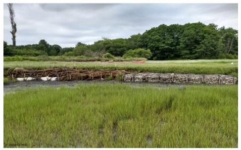
Figure C7. Example of a demonstration living shoreline treatment at an eroding marsh edge that utilizes aged oyster shell placed in coconut-fiber biodegradable bags (left side of image) and plastic-mesh gabion baskets (right side of image). The treatment also beneficially utilizes an in-place tree trunk as toe protection. Image by P. Slovinsky, MGS.
