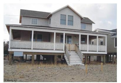
Figure C5. Example of a pile-supported foundation from a structure located in the front dune and within a flood zone. Image by P. Slovinsky, MGS.
