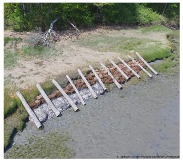
Figure B10. Example of a hybrid living shoreline at Maquoit Bay Conservation Lands, Brunswick, ME, along an eroding marsh edge which beneficially uses woody debris (logs) and integrates biodegradable bags and synthetic baskets filled with aged oyster shell. Image by R. Harbison, GPCOG.
