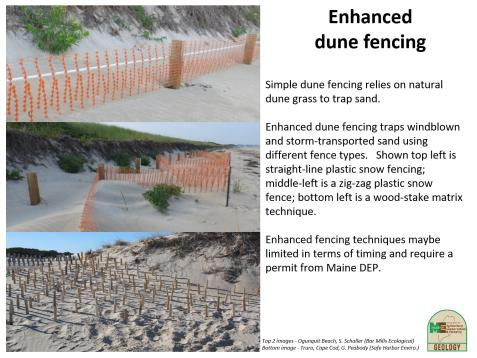
Figure A9. Enhanced dune fencing examples from Ogunquit, ME (top 2 images) and Truro, MA (bottom image). Enhanced techniques are from Bar Mills Ecological (Schaller, 2015) and Safe Harbor Environmental.
