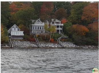
Figure B6. Example of a stable-armored bluff that has been stabilized with coastal engineering structures along the Belfast shoreline. Image by P.A. Slovinsky, MGS.
