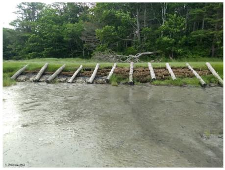
Figure C8. Example of a demonstration living shoreline treatment at an eroding marsh edge that utilizes aged oyster shell placed in coconut-fiber biodegradable bags (center and right side of image) and plastic-mesh gabion baskets (left side of image). The treatment also beneficially utilizes tree trunks to provide protection from winter icing. Image by P. Slovinsky, MGS.
