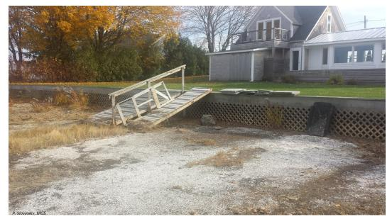
Figure C9. Example of a bulkhead placed adjacent to an eroding marsh edge. Bulkheads generally result in the squeezing out of coastal marshes and limit sediment supply from the upland to the wetland. Image by P. Slovinsky, MGS.
