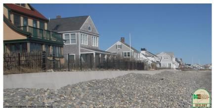
Figure A10. Cobble-trapping fences along Drakes Island Beach, Wells, ME.
